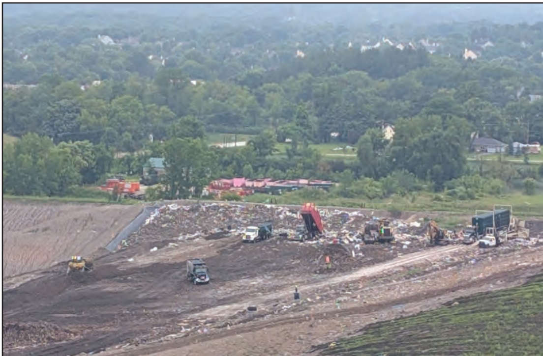
Working face at North end of Phase 4
